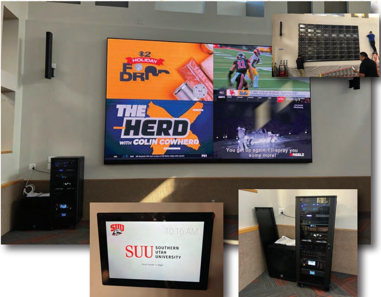
SUU wanted to install a 220" Direct View LED wall inside the Sharwan Smith Student Center lobby. They wanted the ability to configure up to 8 different video sources: 4 Brightsign players and 4 video signals. They wanted to show either picture in picture, or 4 video signals arranged in 2 x 2 - in any way with any of the 8 sources. They also wanted speakers and the ability to provide 2 audio outputs. All of this would be controlled using an Extron touchscreen.
